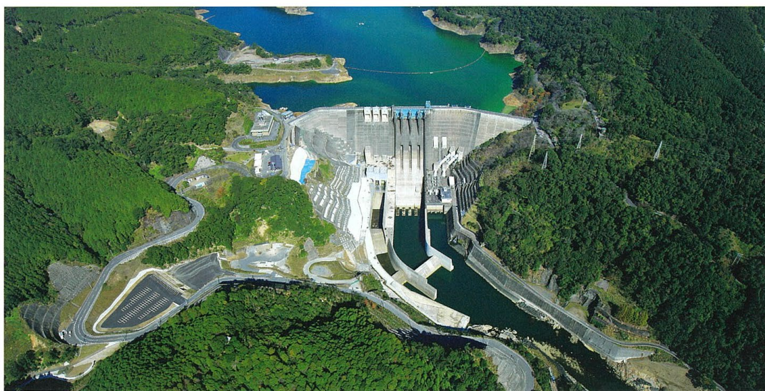
工事完了 Completion of construction
