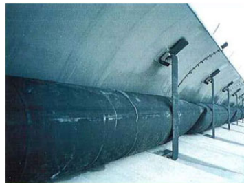
Steel Flap Gate with Rubber Bladders
