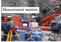
The centralized data management was performed using CIM (Construction Information Modeling) by ground exploration technology, borehole wall observation and so on. It achieved high-accuracy drilling by reflecting the drilling data. Eventually, it enabled more accurate drilling to avoid interference with other underground structures.
