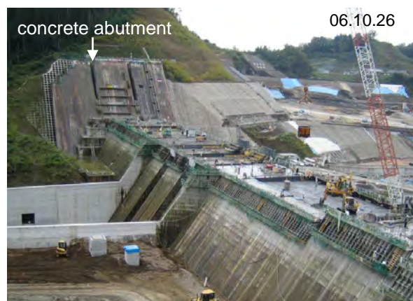
Fig.32 Concrete abutment, Inaba dam
