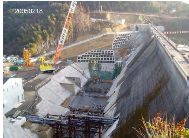
Fig.45 Raising height 5.9m, Shimonohara dam
