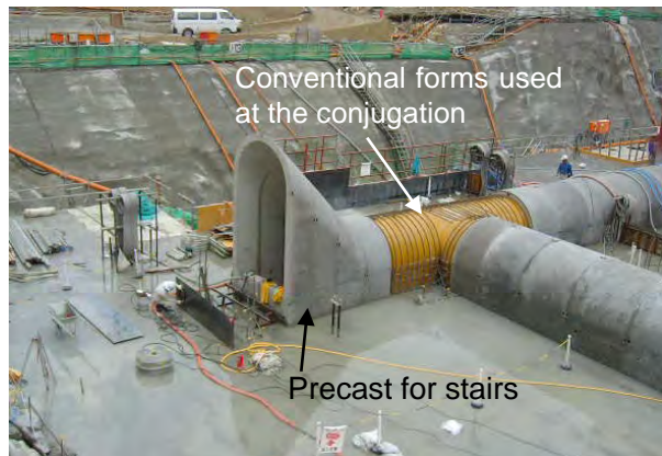
Fig.17 Precast gallery, Kido dam
