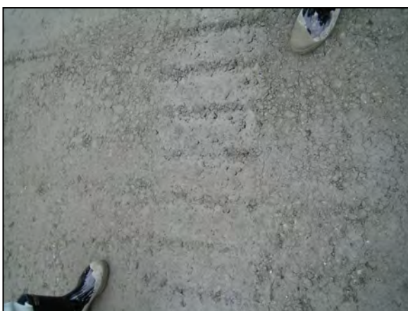
Fig.1 RCD concrete just after compaction
