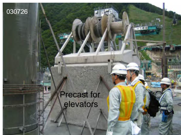
Fig.19 Precast elevator, Nagai dam
