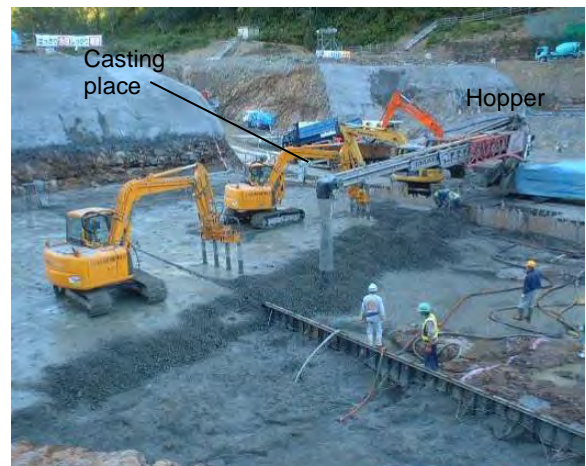
Fig.20 Belt conveyor concrete casting machine with crawler, Toppu dam
