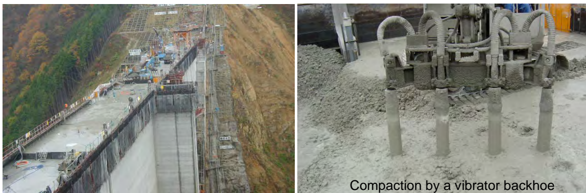
Fig.-13 ELCM (Extended Layer Construction Method), Mimurogawa dam
