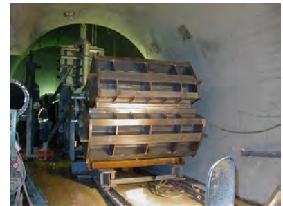
Fig.38 Tension Radial Gate, Haneji dam
