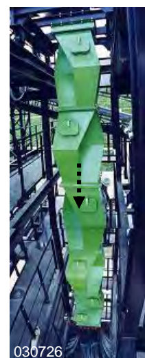
Fig.23 gravity fall mixer, Kido dam
