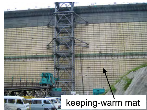
Fig.4 Curing in Nagai dam
