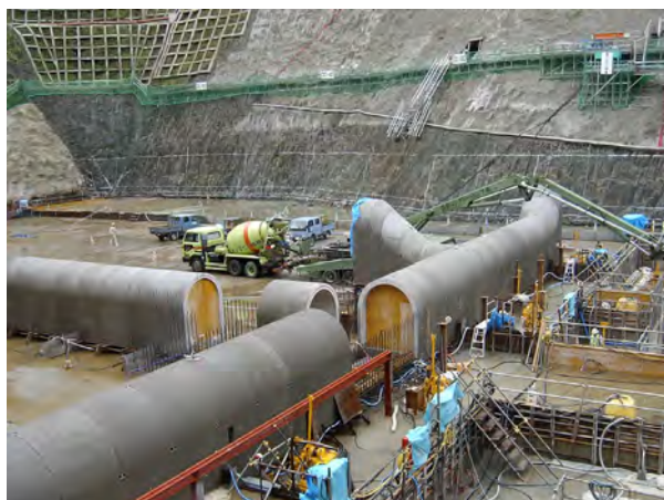
Fig.18 Precast gallery, Hirokami dam
