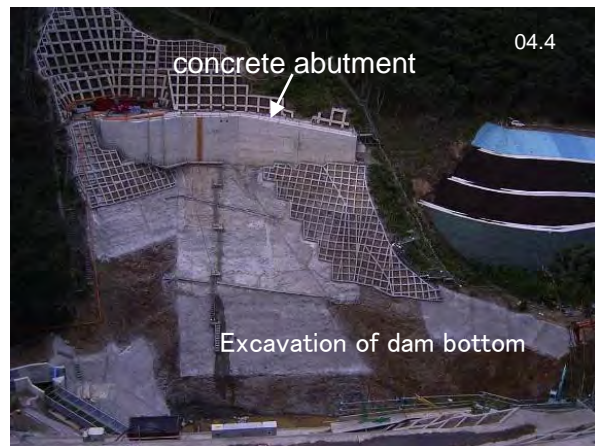
Fig.30 Vertical type concrete abutment , Yamato dam
