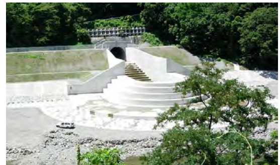
Fig.43 Outlet of bypass tunnel, Miwa dam
