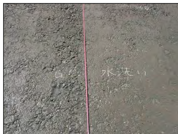
Fig.2 RCD concrete after green cut, wash
