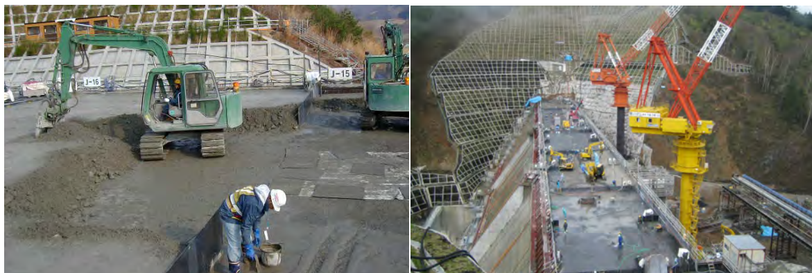
Fig.-14 ELCM, Takoh dam
