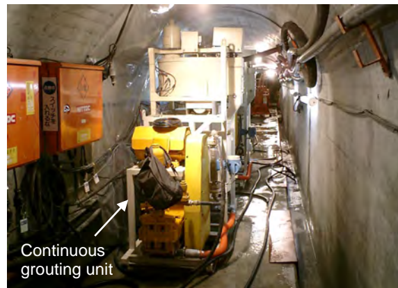
Fig.26 Curtain grouting by a new system
