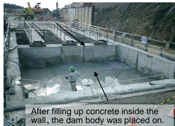
Fig.28 Box type diaphragm, Iwaikawa dam
