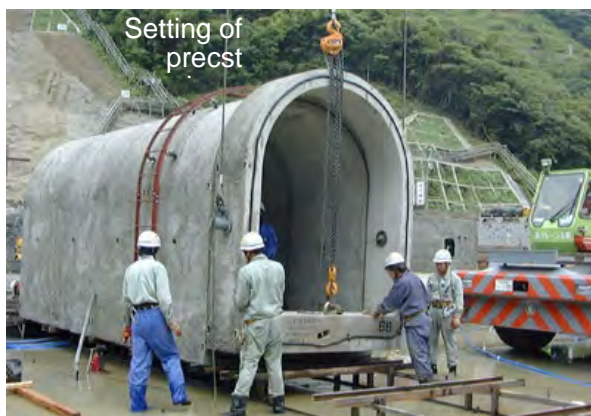
Fig.16 Precast gallery, Fukuchiyama dam
