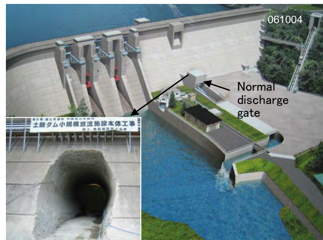
Fig.46 Opening by drilling machine, Haji dam
