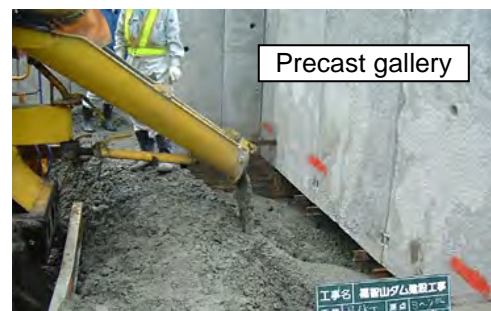
Fig.9 Placement by self compacting concrete (under precast gallery base)
