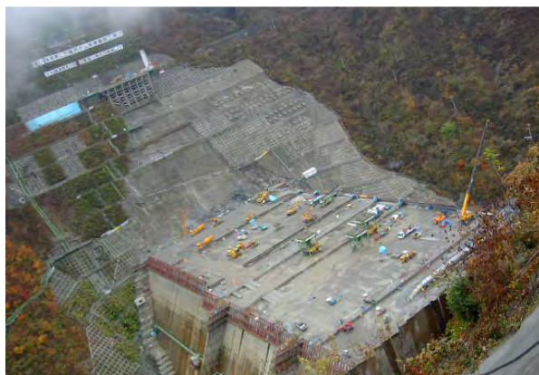
Fig.11 Takizawa dam RCD 021125
